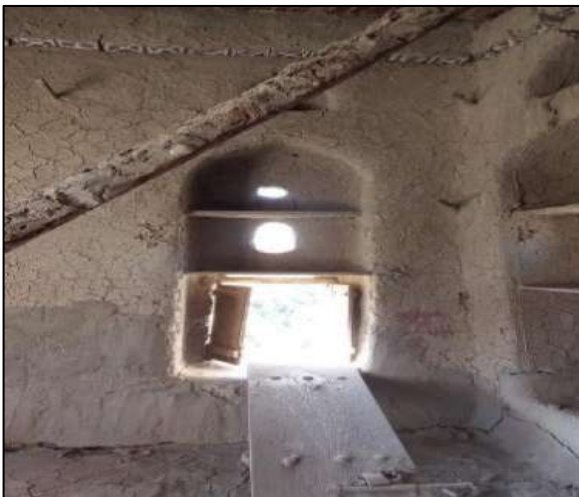
Figure 0.7 Small holes to allow sufficient light and regulate the air in the house at Harrat AL-Bilad, Manah, Oman (2024)
