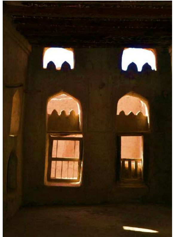
Figure 0.12 Indirect sunlight at the top and body level in a house at Harrat ALBilad in Manah, Oman (2024)
