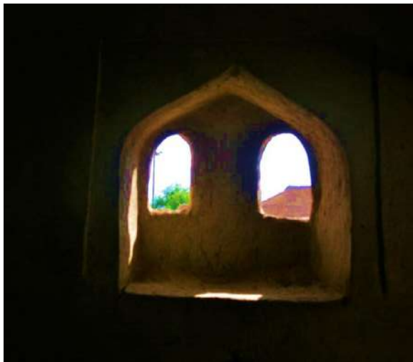
Figure 0.10 Openings in the shape of rounded, triangular, and sometimes rectangular hollows are created to bring in sufficient daylight (2024)
