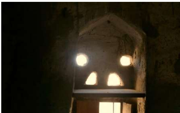
Figure 0.7 Small holes to allow sufficient light and regulate the air in the house at Harrat AL-Bilad, Manah, Oman (2024)
