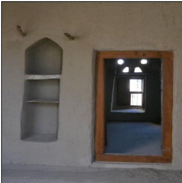
Figure 0.10 Openings in the shape of rounded, triangular, and sometimes rectangular hollows are created to bring in sufficient daylight (2024)
