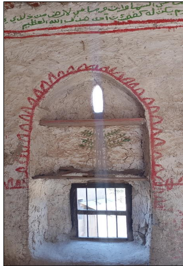
Figure 0.9 High-level small rectangular holes for removing hot air flow purpose at Harrat AL-Busaid, Adam, Oman ( 2024)
